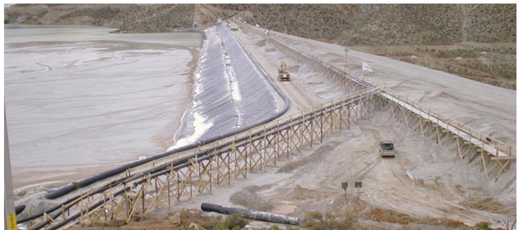
Figure 4. Quillayes downstream sand dam [3]: (a) typical cross-section, and (b) upstream geomembrane.
