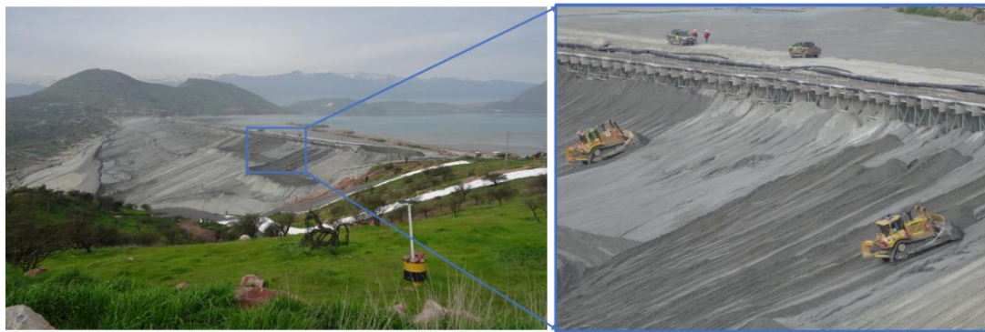
Figure 3. Las Tórtolas downstream sand dam [3]: (a) typical cross-section, and (b) flattening and compacting the downstream slope.
