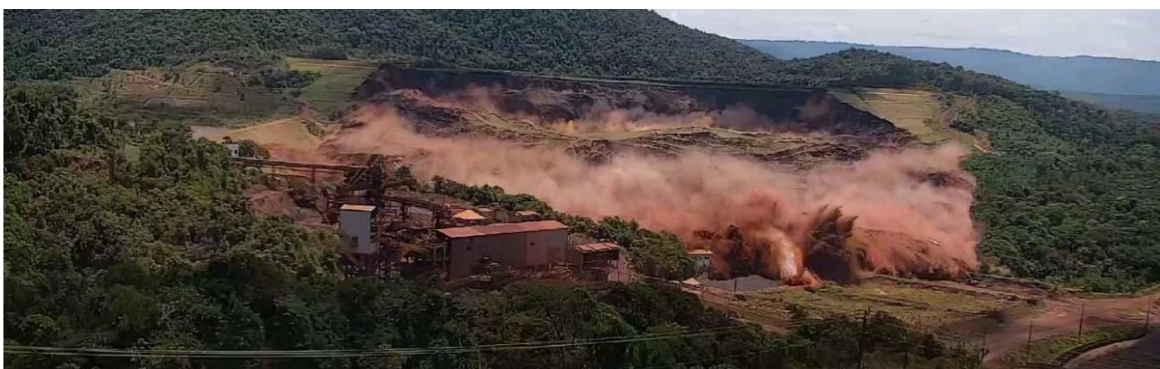
Figure 9. Failure of Feijão tailings dam I due to rapid flow liquefaction [10].
