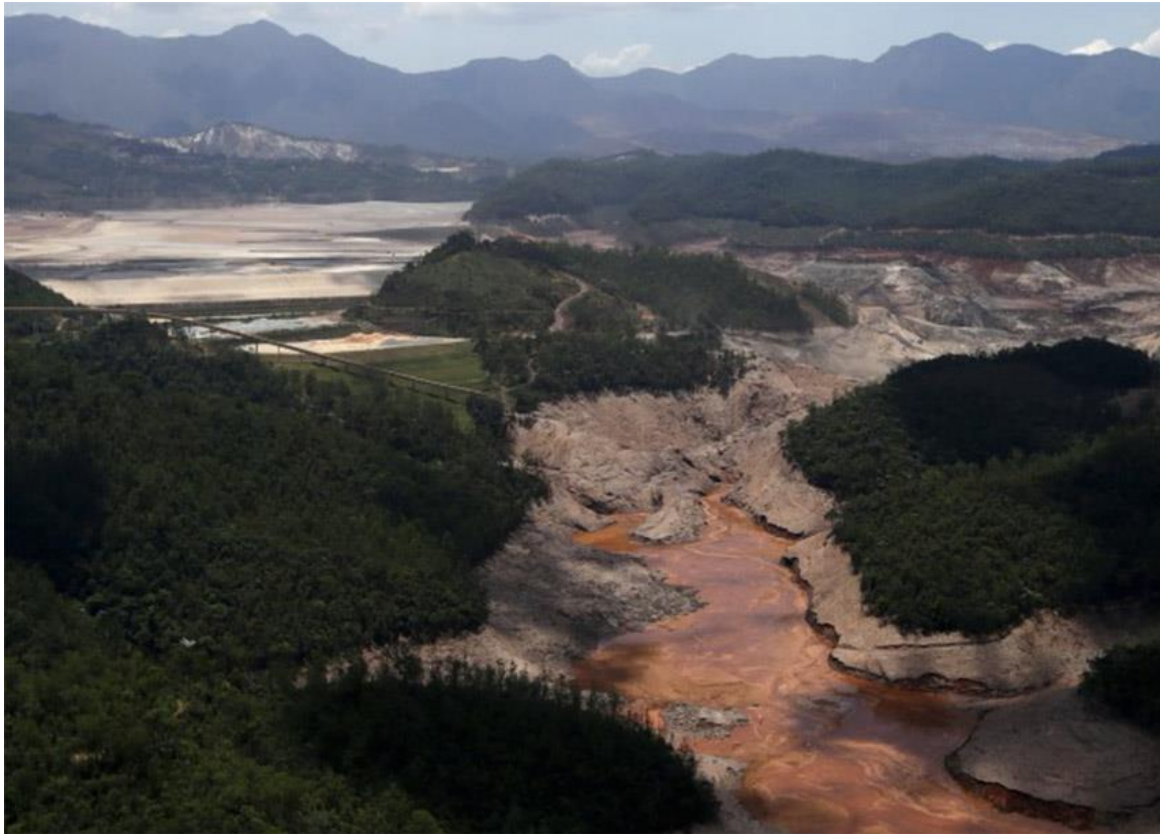
Figure 8. Failure of the Fundão tailings dam due to rapid flow liquefaction [9].
