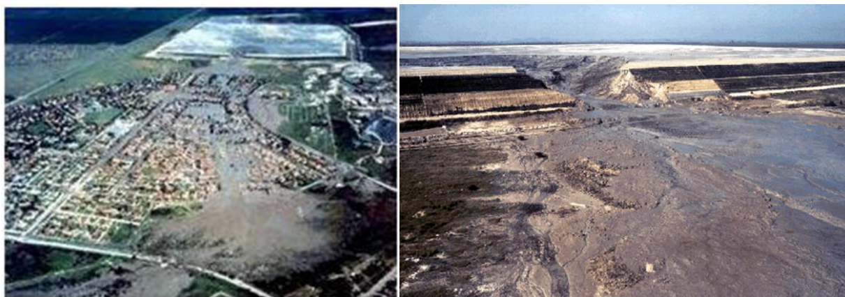
Figure 5. Failure of the Merriespruit tailings dam in South Africa, due to overtopping and flow liquefaction [5].
